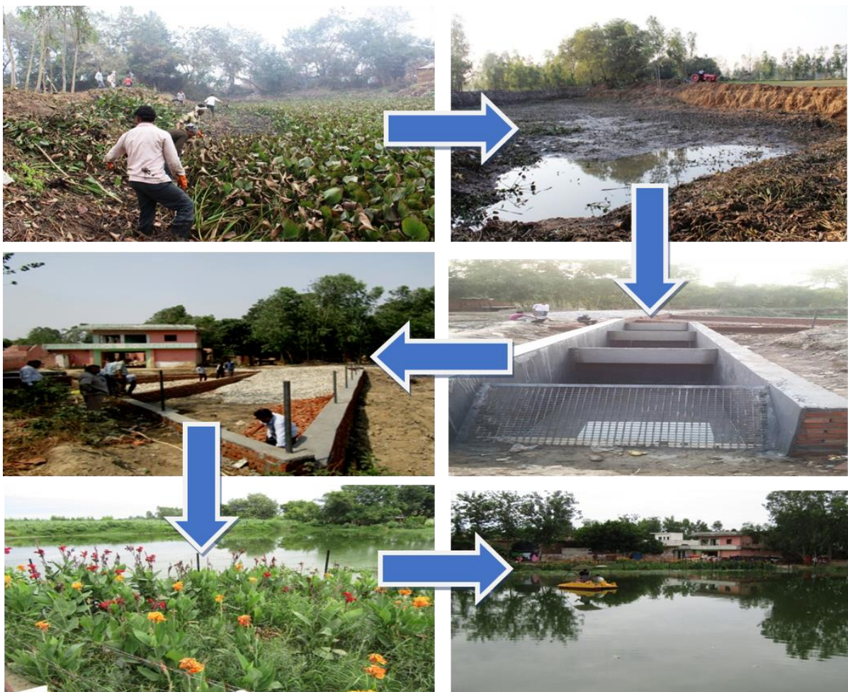
Fig. 4a: Pond Rejuvenation and establishment of CW-NTS at Ibrahimpur Masahi pond
